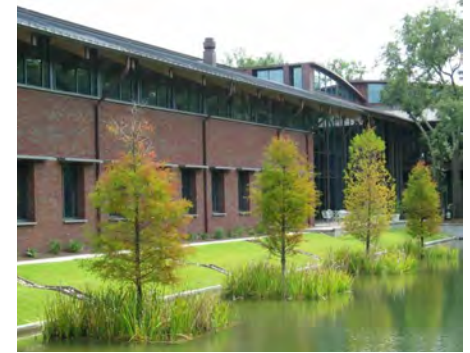
Constructed wetlands used to purify water.
